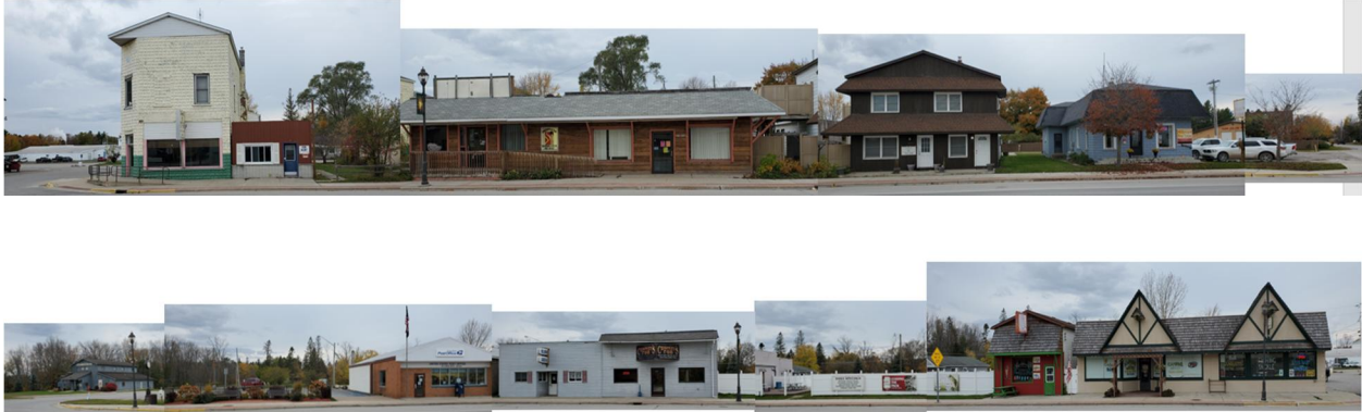
Examples of breaks in the building walls in downtown
