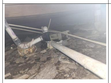
Photograph shows a closeup of one of the sanitary lines. No suspect materials found.
